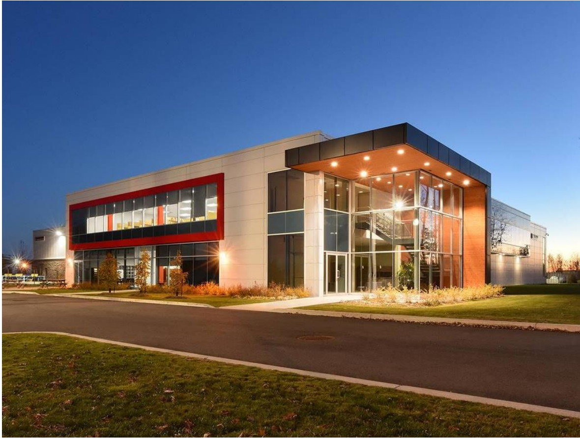
Urecon, Coteau-du-Lac (Quebec, Kanada)
